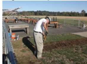
8-15 Trench for underground sprinklers
