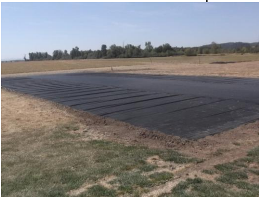
8-25 Trenched dug out and geotext stretched
