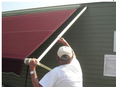
9-8 Club house awning repair - East Brace lock seized, replaced with new (both)
