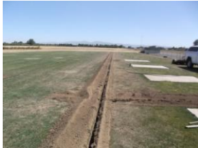
8-15 Trench for underground sprinklers
